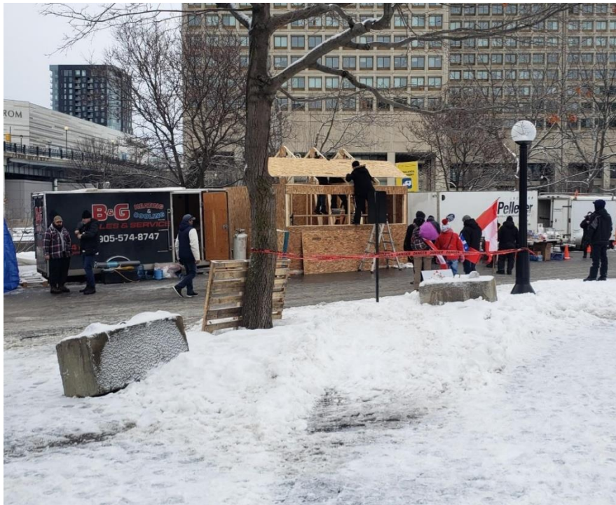
Construction of wooden shed at Confederation Park 55
