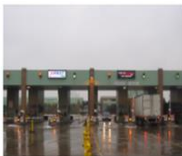
Commercial vehicle primary inspection lanes (PIL)
