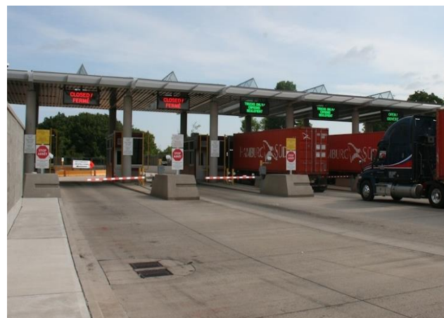
Queenston Bridge – Commercial primary inspection lanes (PIL)
