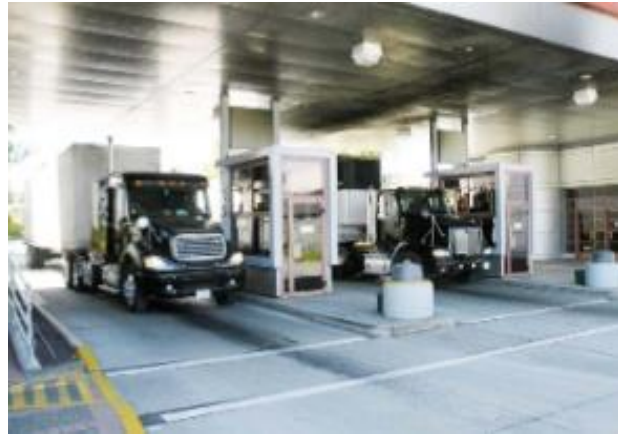
Pacific Highway (commercial) port of entry, primary inspection line (PIL)
