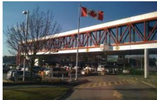
Pacific Highway (traffic) port of entry, primary inspection line (PIL)
