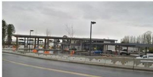
Aldergrove port of entry, primary inspection lane (PIL) and secondary area
